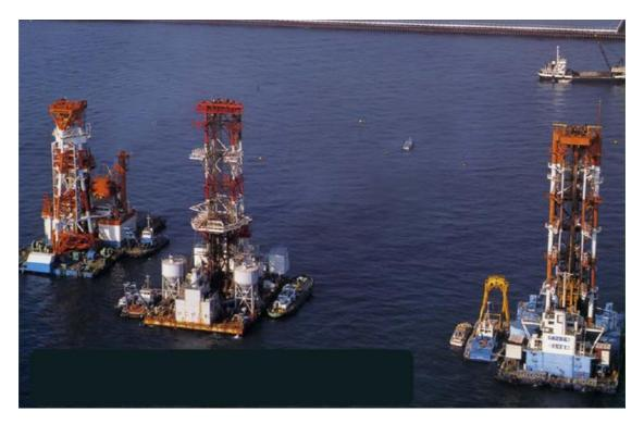
Figure 5.34 : Land Formation by Deep Cement Mixing (DCM) Method
